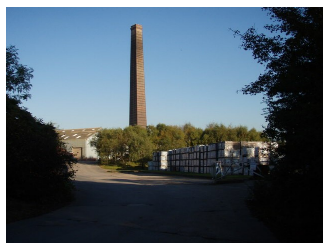
The chimney, a local landmark.
